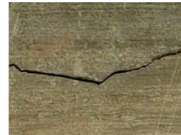
Fig.2 Image awaiting repair 图2 待修复图
